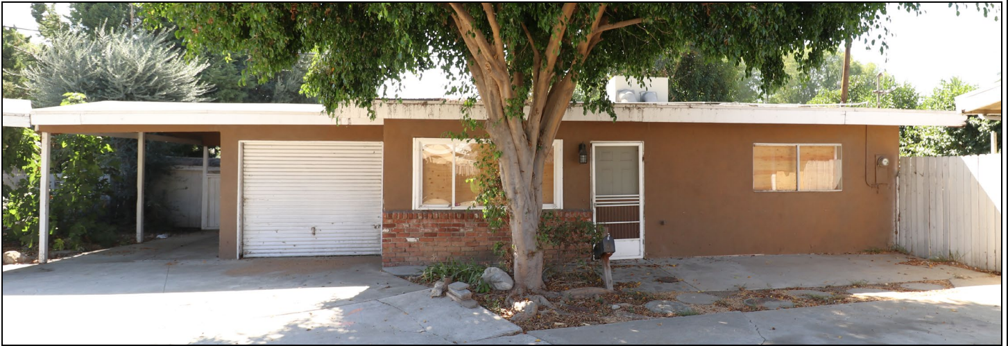
2677 A Street, façade, view south (10/8/24).
