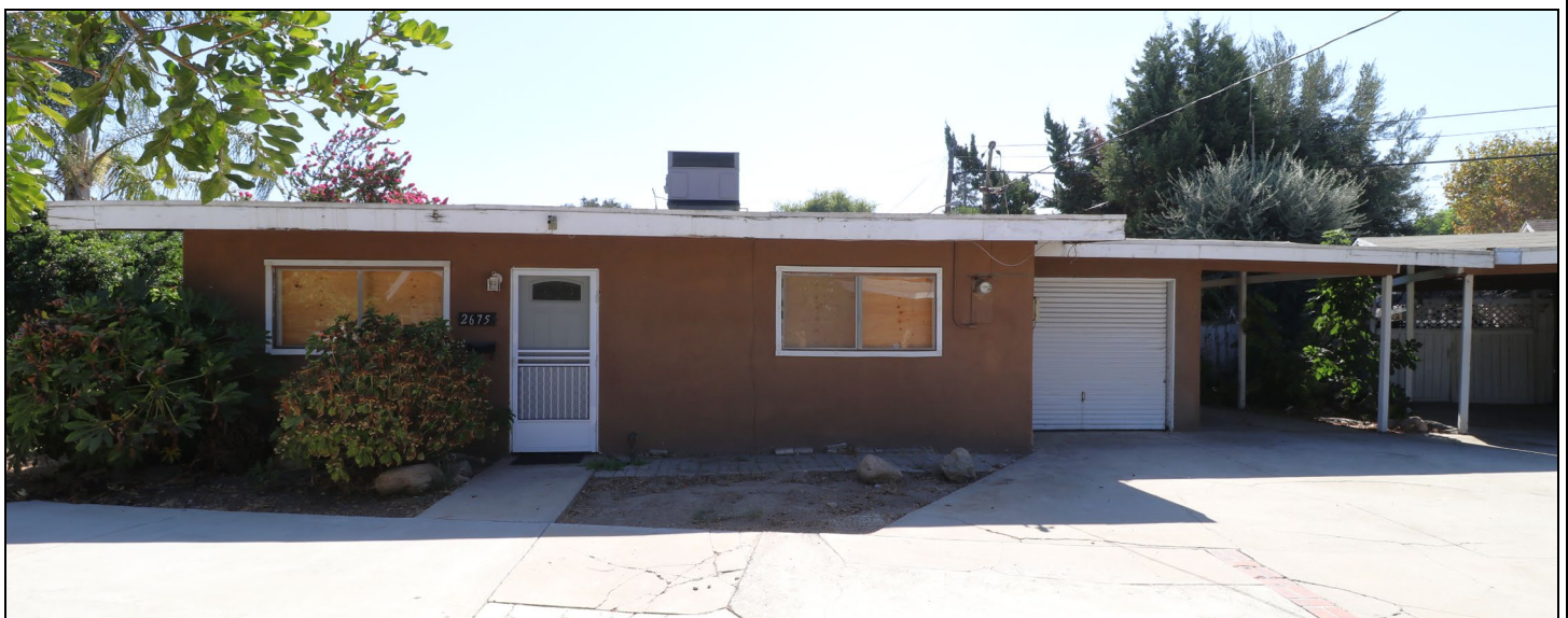
2675 A Street, façade, view south (10/8/24).
