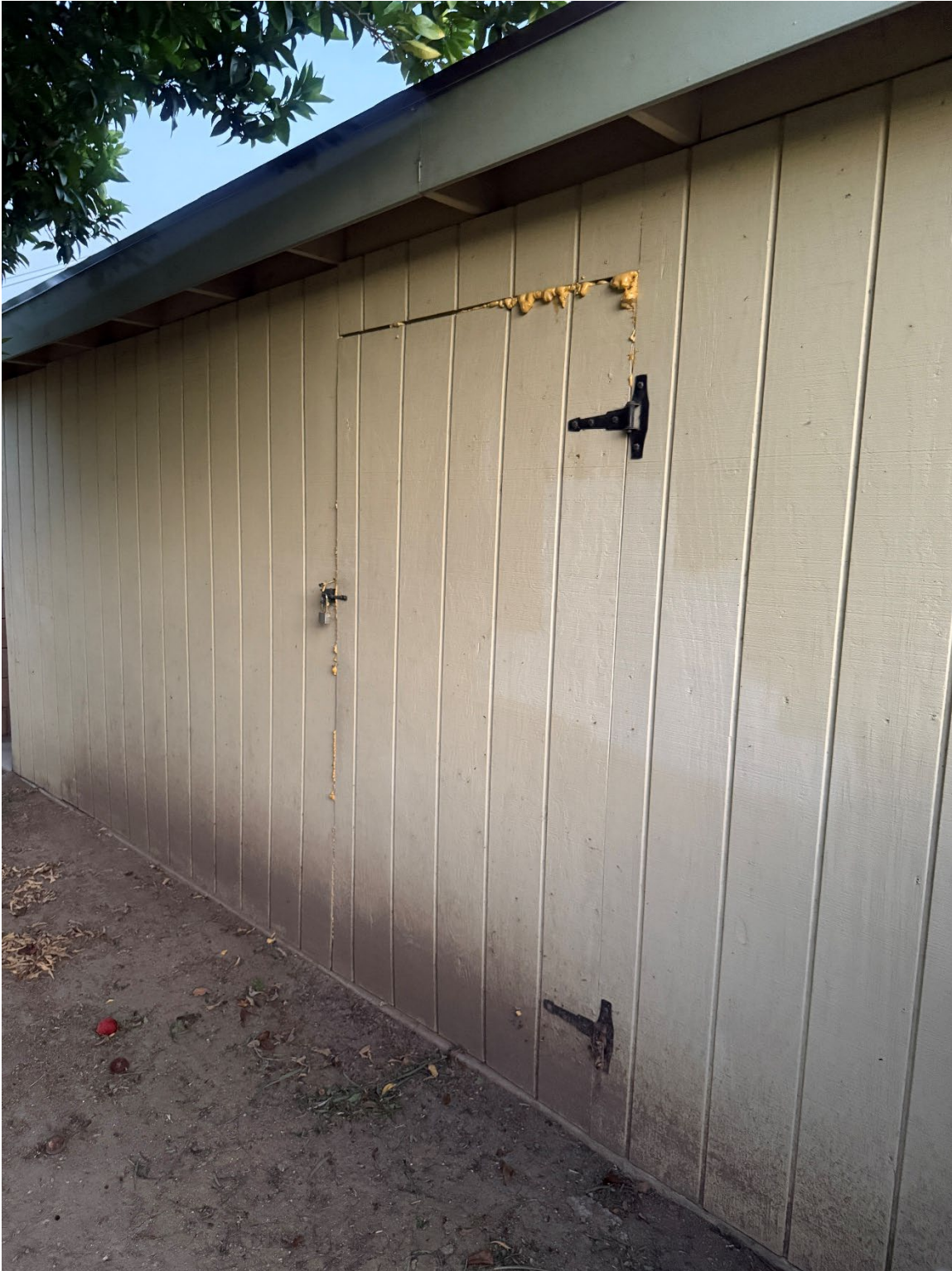
Figure 4 – Door exclusion with spray foam
