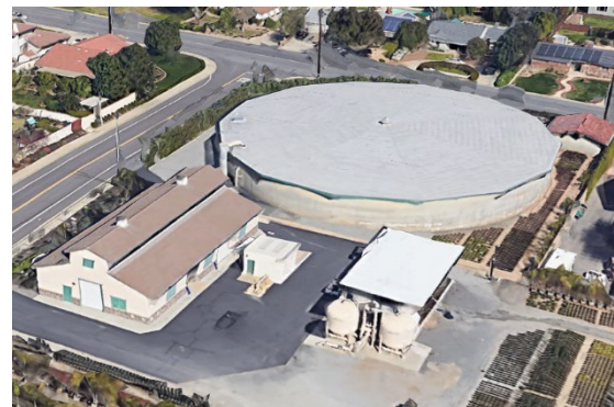
Amherst Booster Pump Station
