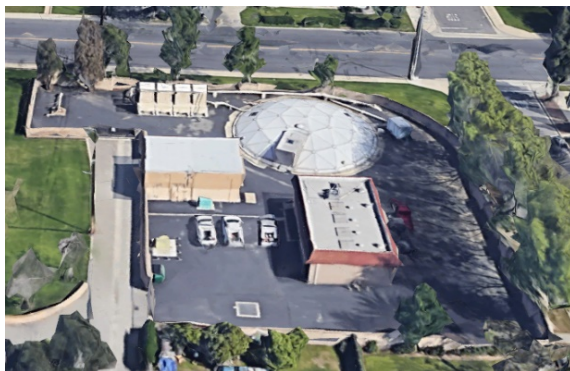
White Avenue Pump Station
